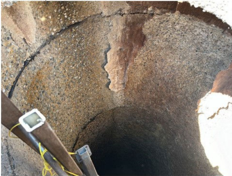
Photo 4. Gravity Line Manhole.
