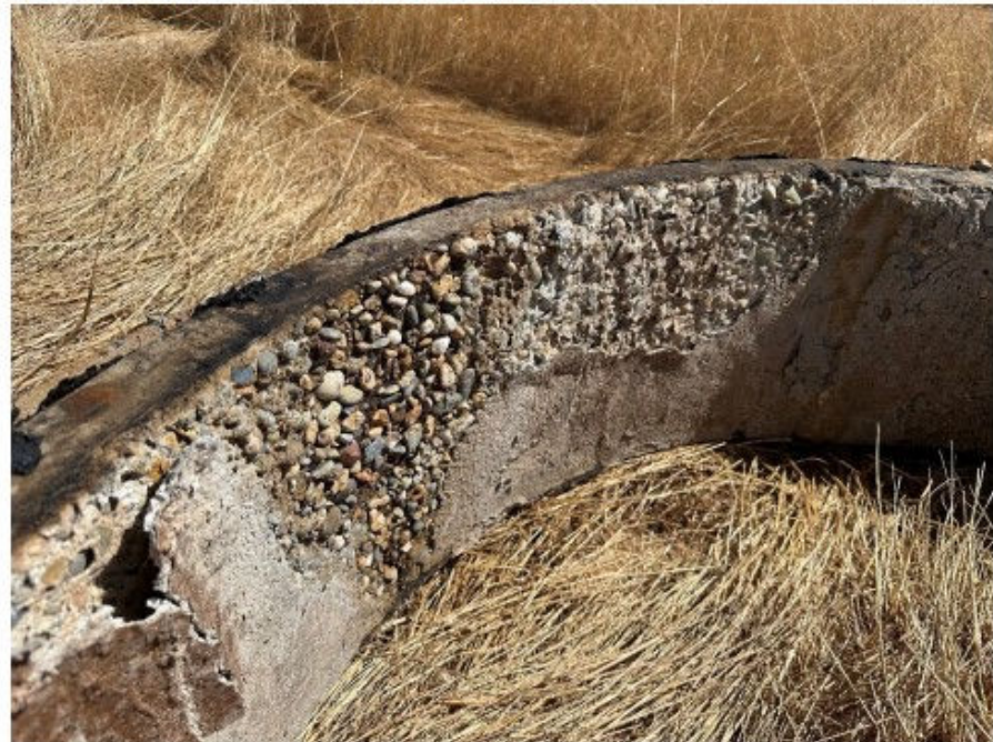
Photo 5. Barrel section removed from manhole.
