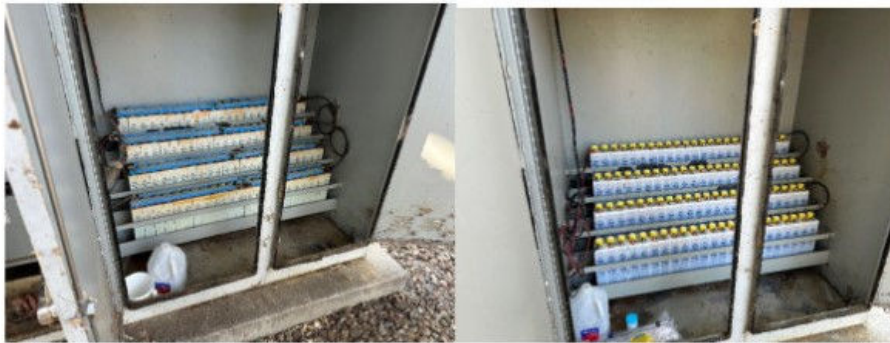
Photos 3 & 4 Old and new Main Switch Gear breaker battery charging system.
