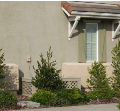
ENCOURAGED: AC units are screened from view by low fencing and landscaping
