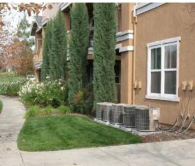
NOT PERMITTED: AC units are located next to building entrances and not screened from view.
